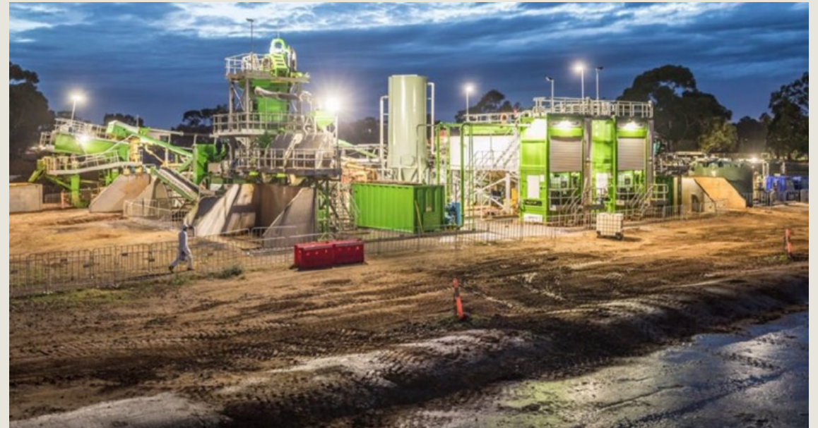
A full scale PFAS-impacted soil washing plant in Australia
