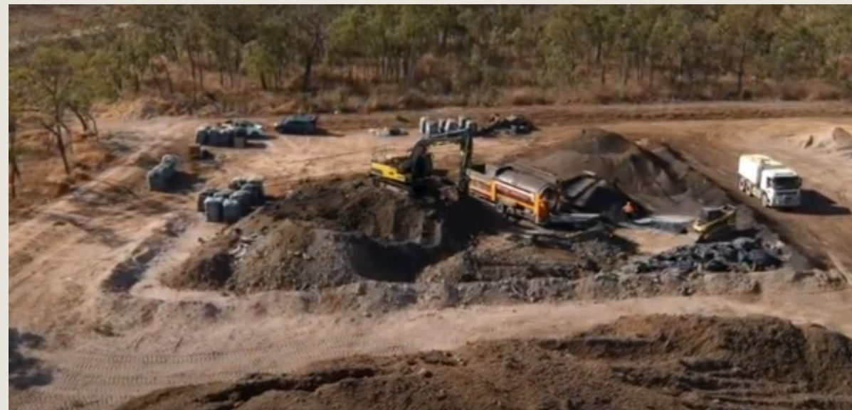
A full scale PFAS-impacted soil stabilization project at a military base in Australia. Image courtesy of RemBind™
